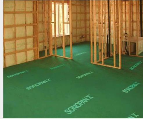
**SONOpanX® flooring acoustic panels are effective, light and easy to cut and install.**
